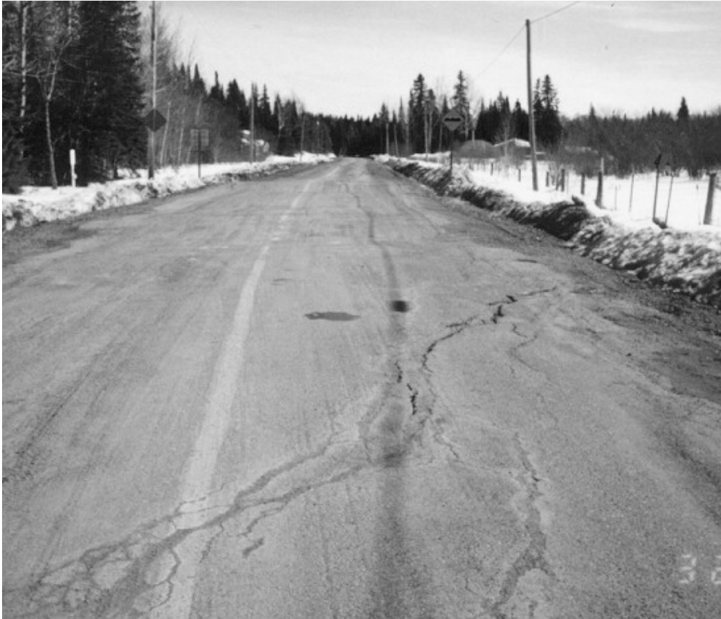
Figure 5 Differential Heaving of a road within a pipeline ROW
