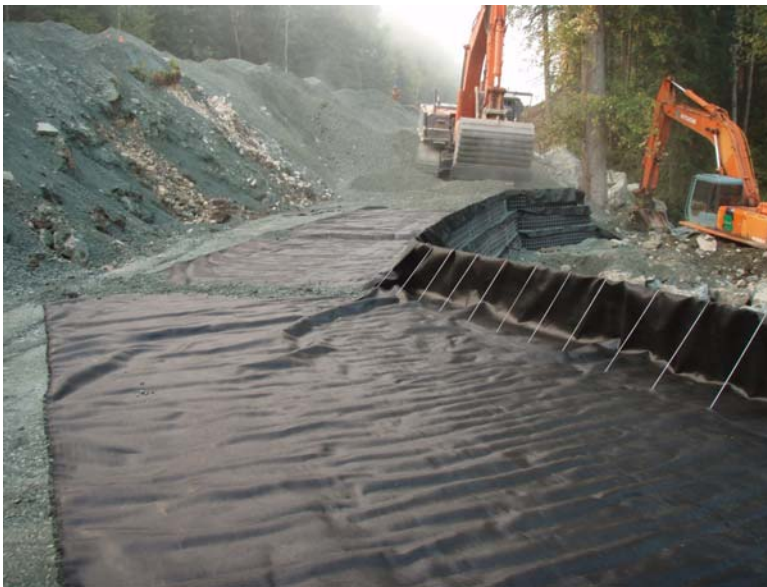
Figure 10 – Matheson Siding: Starbaby Creek Looking Track-north Illustrating Wall Geometry and GRS System.
