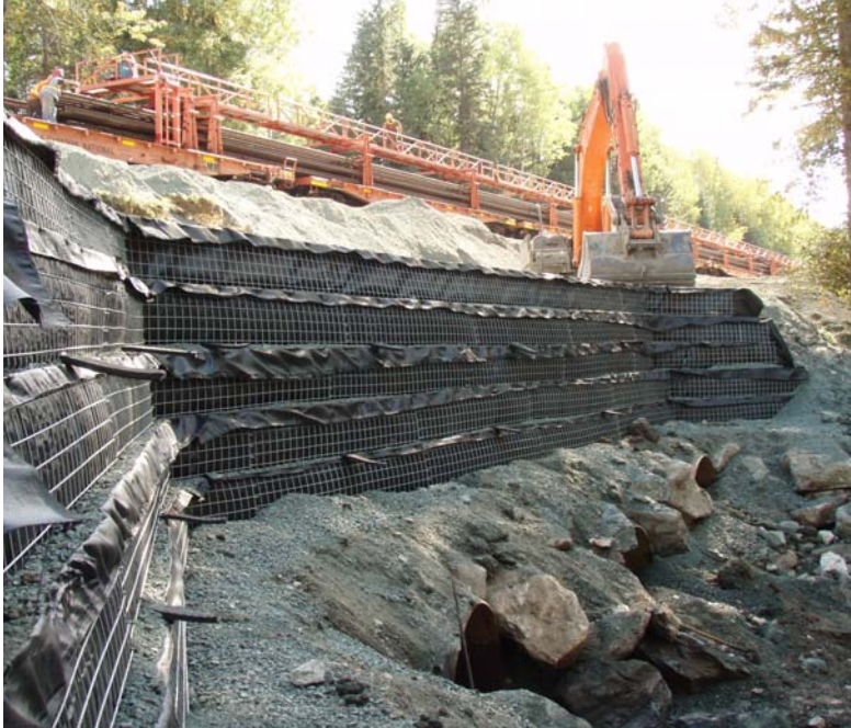
Figure 12 – Matheson Siding: Bittner Creek. Typical Section at Culvert and View Looking Track-north at Completed Wall. Note Zero Encroachment on Riparian Zone at the Pre-Existing 9 ft Wide by 6 ft (2.7m x 1.84m) High Concrete Box Culvert Outlet. System Facing Weld Wire Mesh Form Height is 1 ft 10 inch (0.56m) per Form. Geotextile Spacing is 11 inches (0.275m). All dimensions are in metres.
