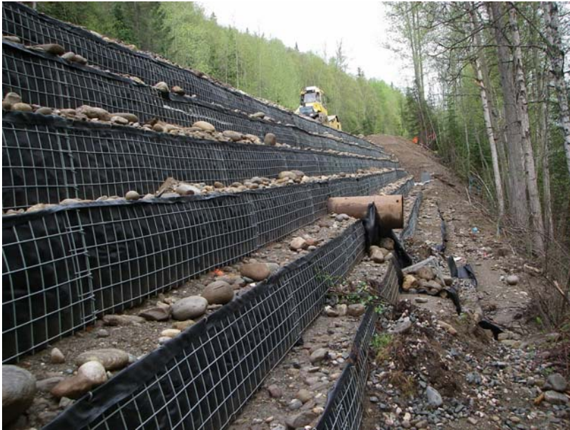
Figure 5 – Poser Siding: Wall 1 – View Looking Track-north at Completed Wall.
